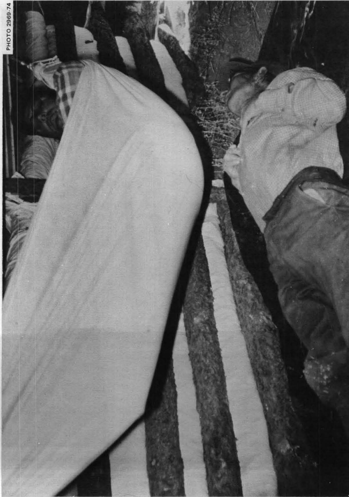
Fig. 4.31. Using an expedient Bedsheet-Hammock, to enable two persons to sleep over the same floor space. Otherwise, only one person could sleep in this space in an Above-Ground Crib-Walled Shelter. The ceiling was only 40 in. above the floor.
